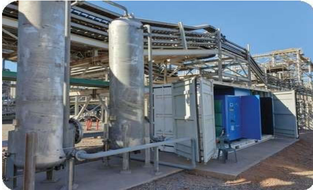
Containerised compressor packages, purpose-built for dusty, high-heat mine environments.
